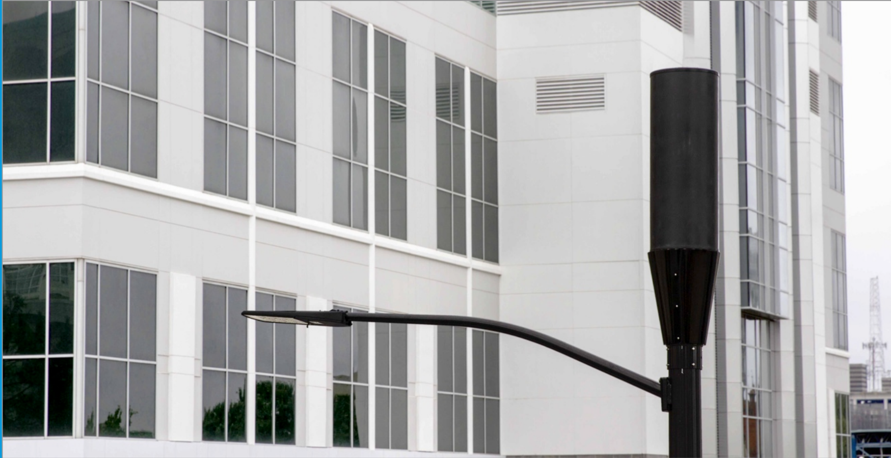
Camouflaged Antenna on Streetlight
